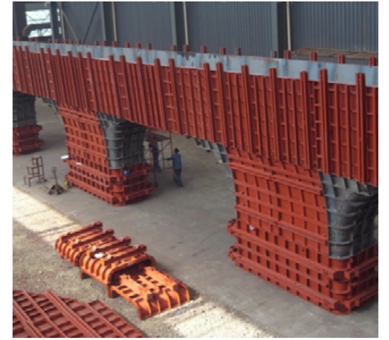
Steel Formwork Support System for Bridges 桥梁钢模支撑体系
