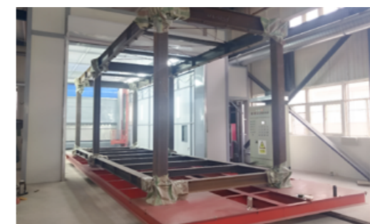
Rust Removal, Painting 除锈、喷漆
