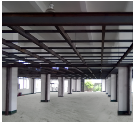
Steel Structure Mezzanine 钢结构夹层
