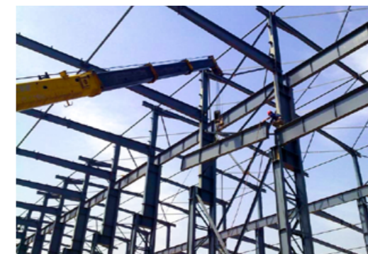
Light Steel Factory Building 轻钢厂房
